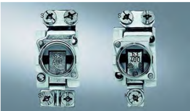
NEOZED base with: K = screw head contact S = saddle terminal
